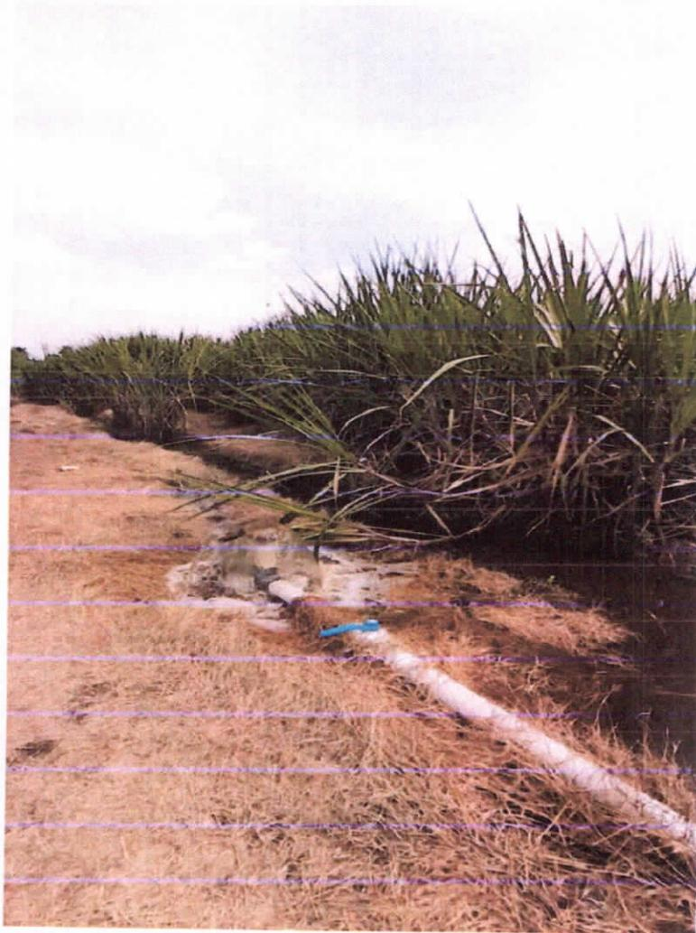
*Treated effluent discharge in agricultural field through pipe line*
